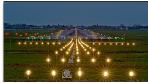
Typical Approach Lighting System (FAA)
